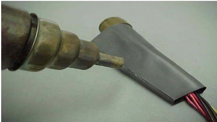
Photo 5 Shrinking tubing using a reducer nozzle.
