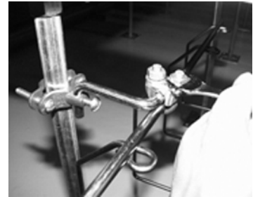
Fig. 5 Securing the 201 Series Snake Tray under an access floor to the vertical pedestal base using the ST-201 bracket.
