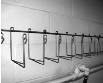
Fig. 6 Wall Snake attached directly to the wall using CM-501-CA anchor bolts
